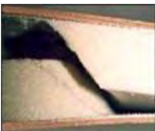
Typical shear failure shown with foam cored sandwich panel.
