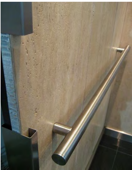
Plastic Honeycomb cored natural stone panel in commercial elevator installation.
